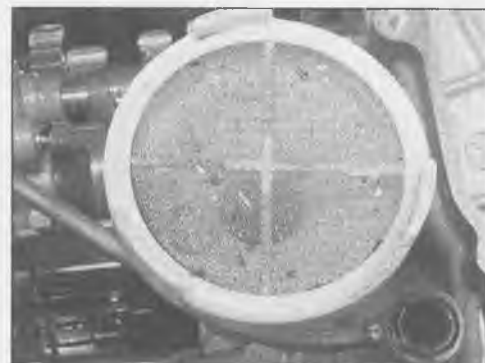
16.7a Inspect the screen on the oil pick-up tube for signs of engine damage
