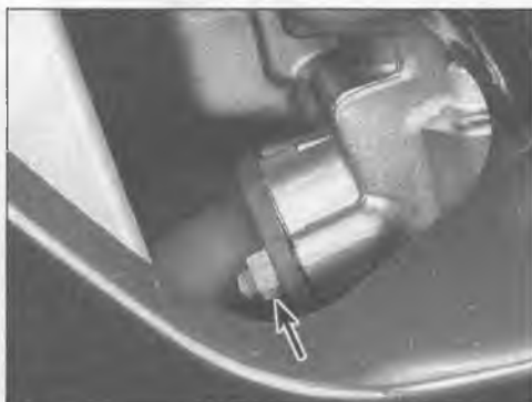
18.5 The exhaust pipe flange nuts (arrow) should be checked frequently and tightened if necessary
